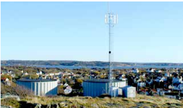
Newly acquired Air-Site AB's free cooling products use nature's own forces (the low impulse principle) for climate control. Customers get even, comfortable temperatures all year round, which helps save a lot of energy. The company has been a green technology pioneer, and by working with big companies like TeliaSonera and Ericsson, they developed the most efficient energy saving solutions on the market, which are now a given by telecom operators.
