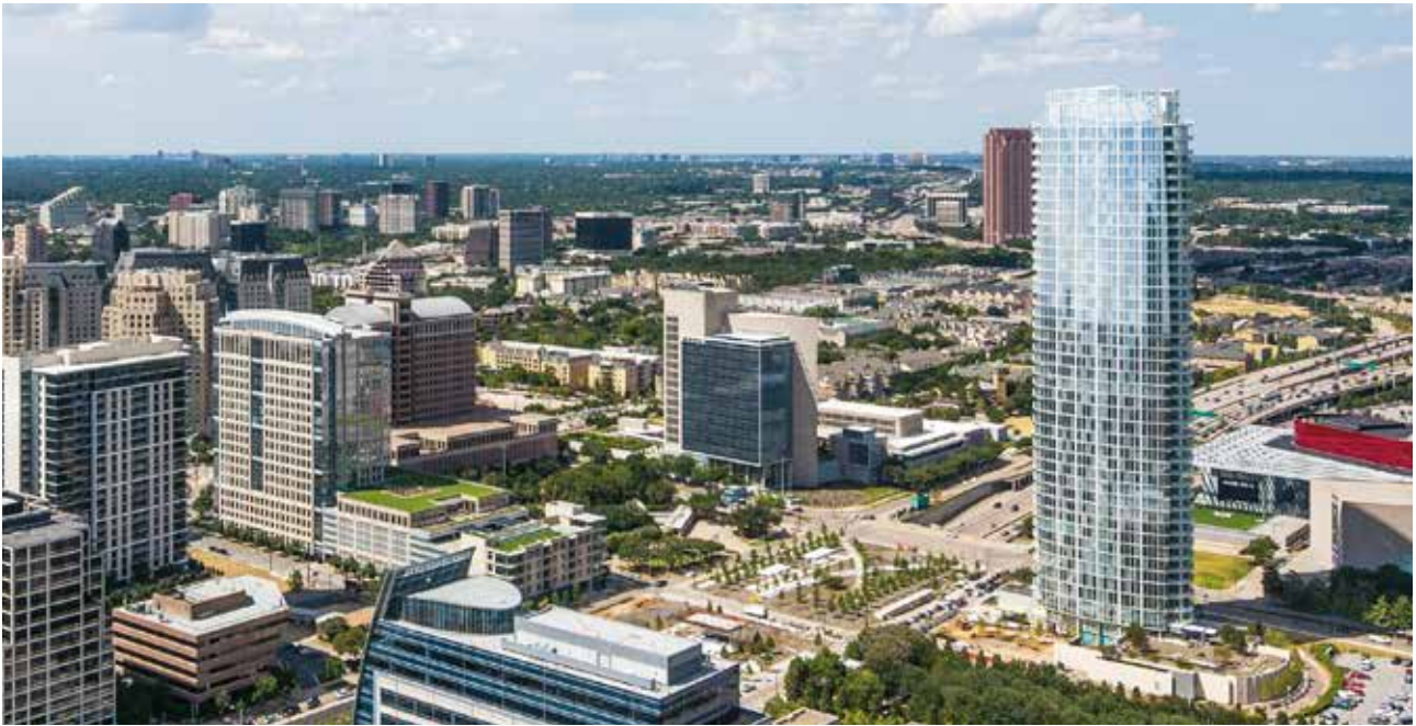
Museum Tower is the tallest residential building in Dallas. With its modern architecture, it is a unique and attractive residential property. The construction consortium chose ClimateMaster to supply the heat pump system for the entire building. ClimateMaster is the best known brand of the recently acquired Climate Control Group, the leading manufacturer of HVAC solutions for commercial buildings and detached homes on the North American market.
