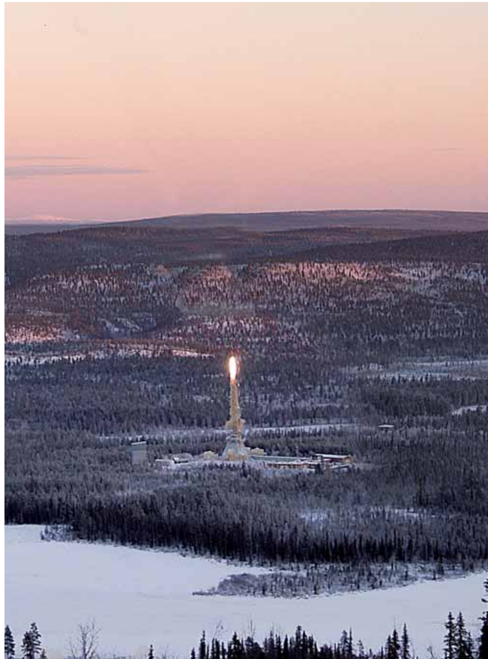
The Esrange Space Centre in Kiruna in the Swedish Arctic heats all 97 of its hotel rooms with NIBE heat pumps all year round.
