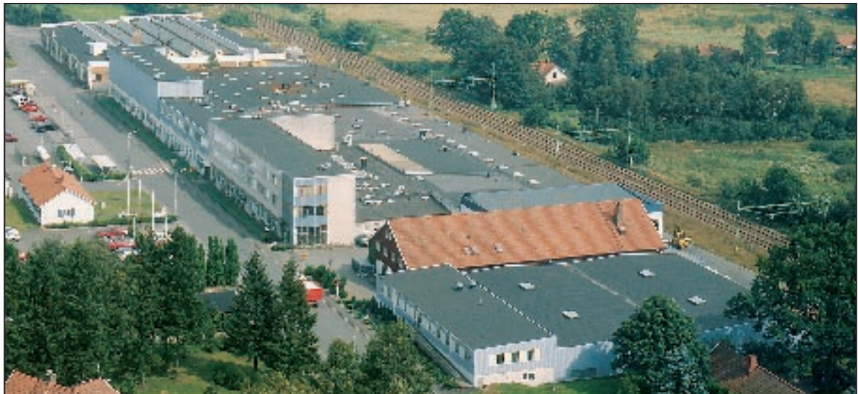
Backer Elektro-Värme AB in Sösdala, southern Sweden.
