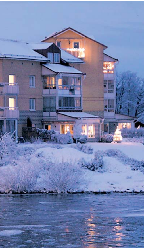
Geothermal pumps can dramatically reduce the amount of energy consumed by large properties.
