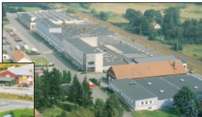
Backer Elektro-Värme AB in Sösdala, Sweden
