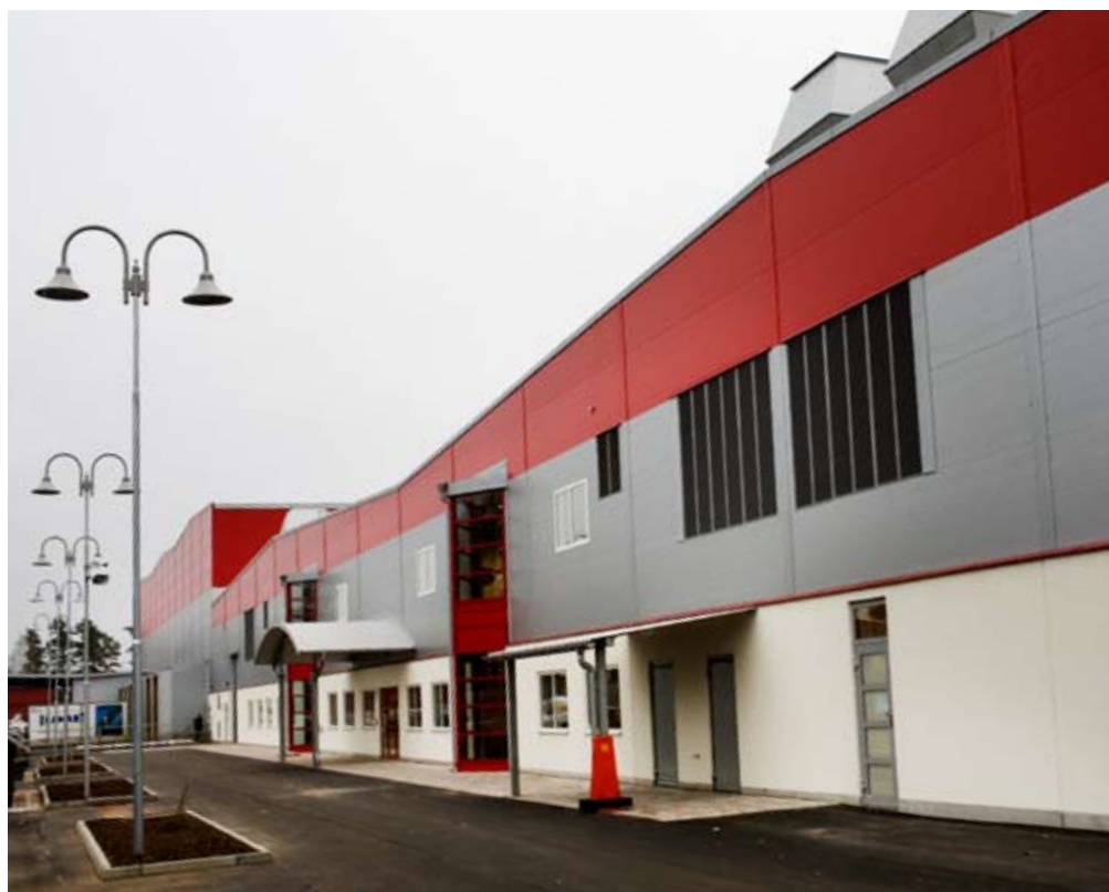
The new stove production plant built in Markaryd in 2007 and brought into use in 2008 represents a major investment in highly automated manufacturing in Sweden.
